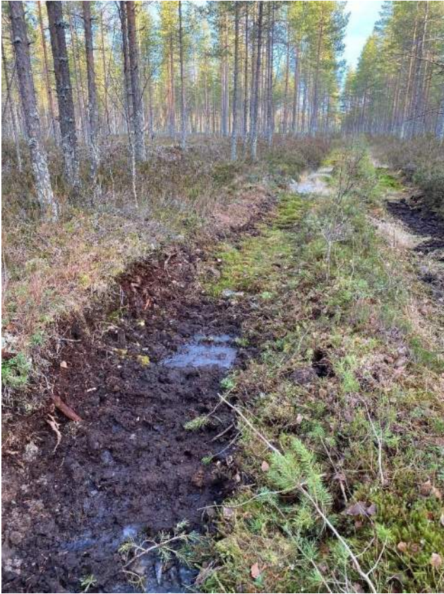
Figure 16. Coarse sand is widely exposed to the power line construction site.
