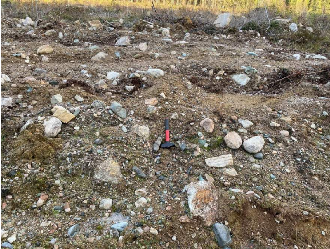
Figure 13. Sandy till in the power line construction site.
