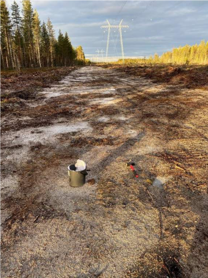
Figure 15. Coarse sand is widely exposed to the power line construction site.
